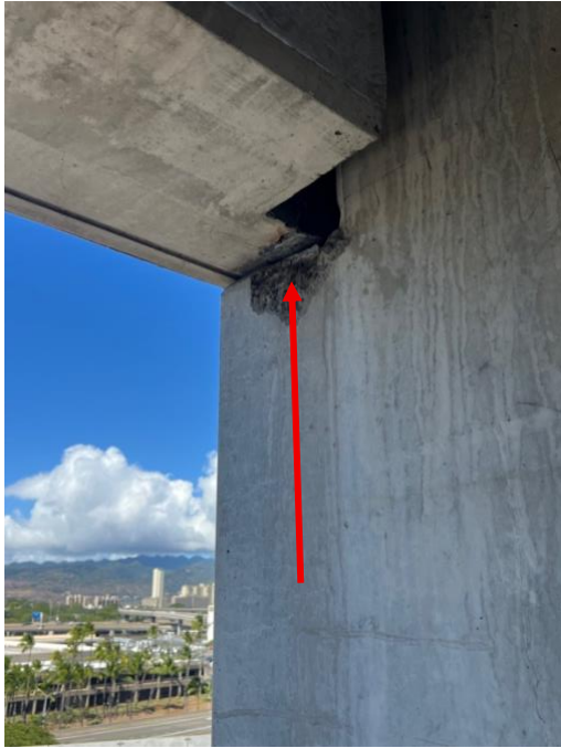
No asbestos detected in tested Vertical Support Pillars
