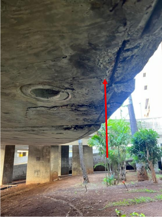
No asbestos detected on the underside of Terminal 1 Parking Garage Freeway Viaduct
